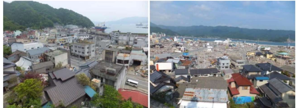
Damage from the tsunami inundation of Kamaishi city with a maximum runup height of 11.7 m (1/6/2011) and of Ofunato city with a maximum runup height of 10.9 m (1/6/2011)
