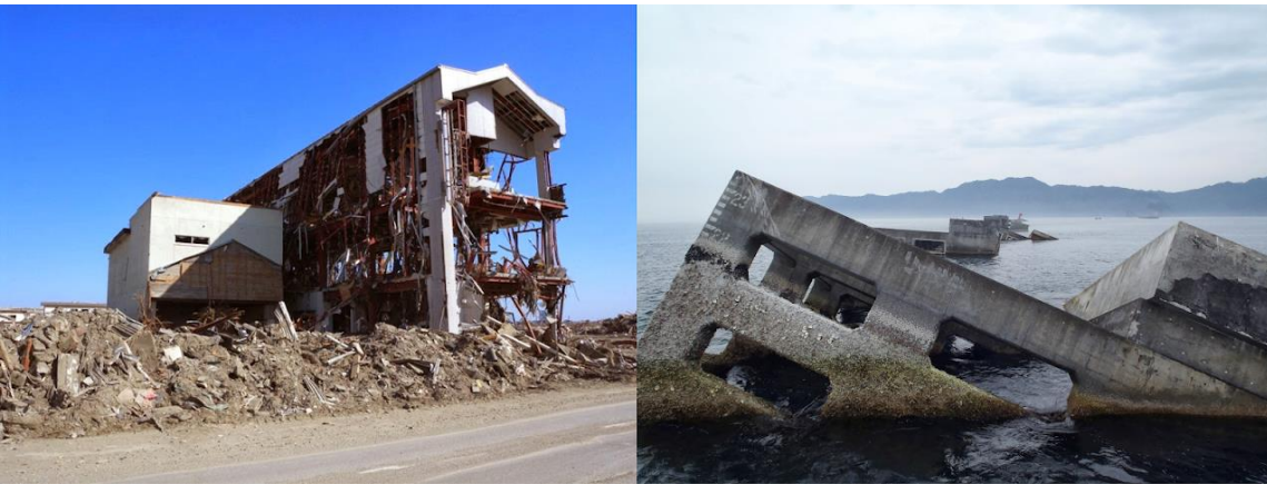
Coastal damage observed in 2011 Tohoku tsunami
