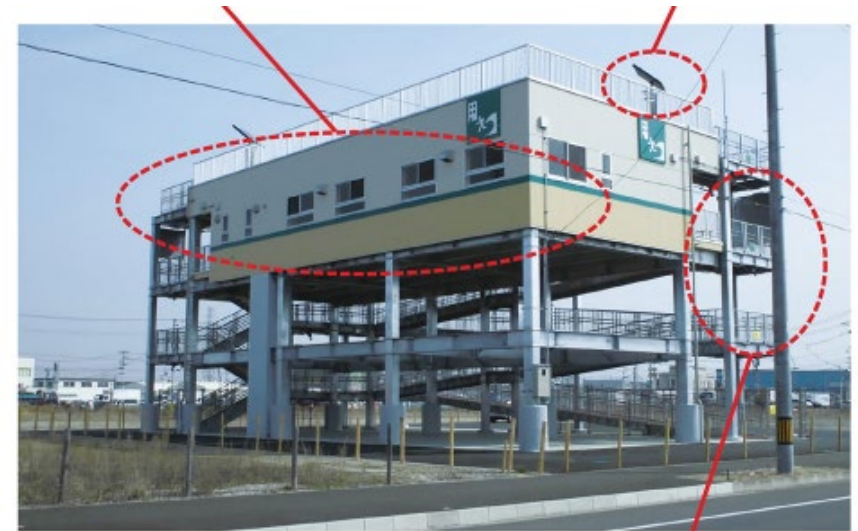
▲ Tsunami evacuation tower
